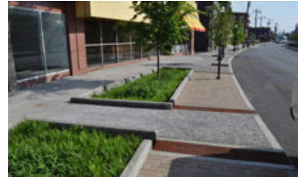
Biofiltration on the sides of streets in an urban area.
