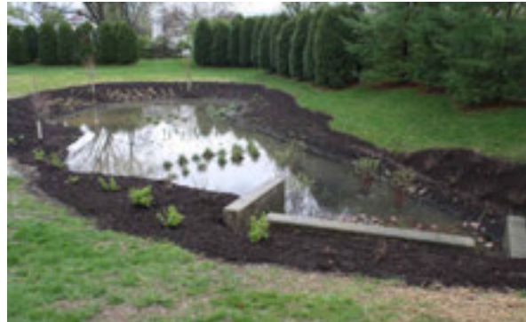
Rain-gardens help manage stormwater in suburban and urban areas.
